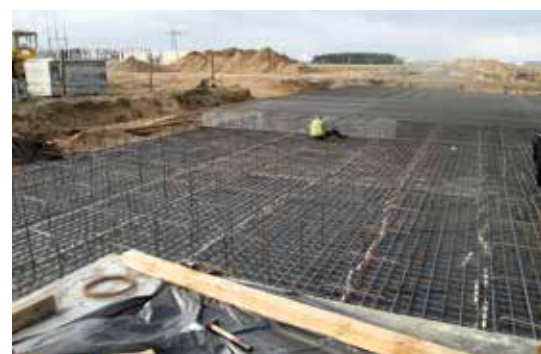
Fundament kottowni
